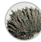
scaling in the boiler
